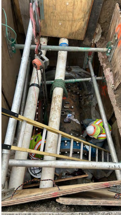
Figure 1 – Installation of Refurbished 24” FW Valve.
