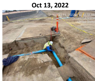
6" Water Line Relocation
