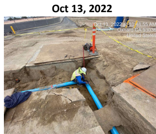
6" Water Line Relocation
