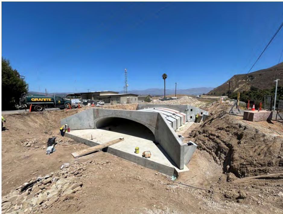
Figure 7 - Granite backfilling and sealing new precast structure.
