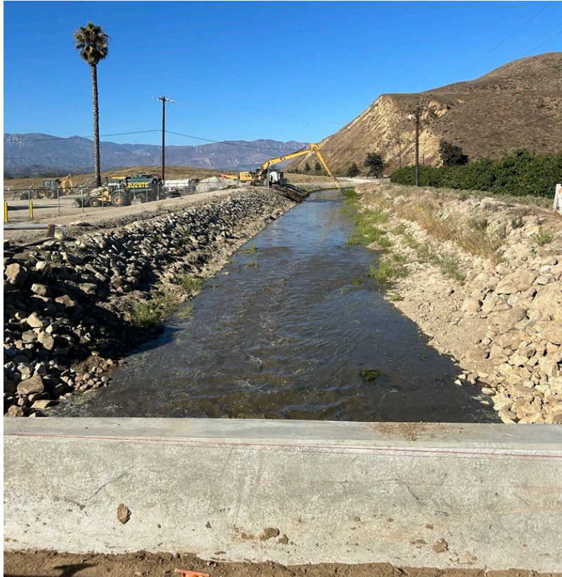
Figure 1 - Water flowing under the new bridge (Inverted Siphon Replacement)
