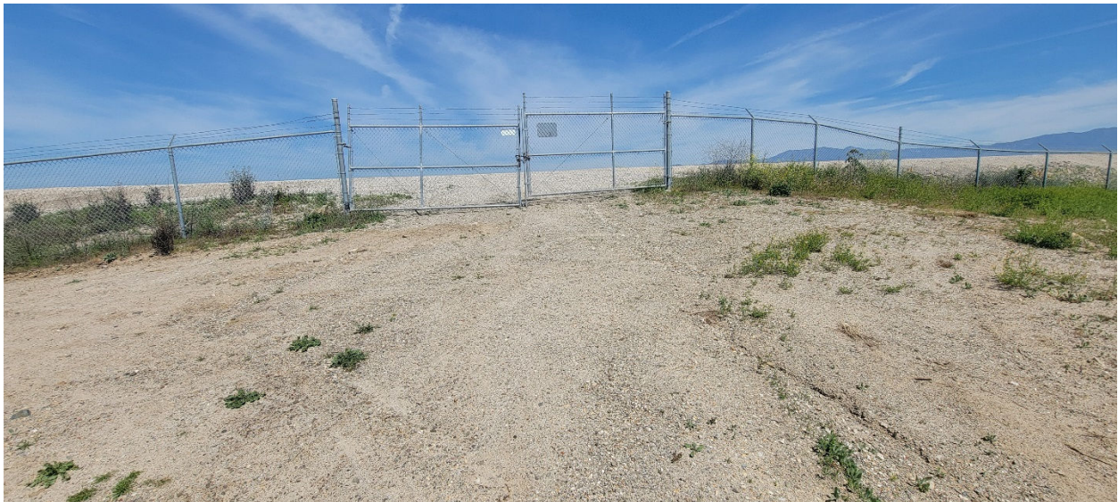
Figure 4 The Santa Clara River Levee Observed from the Western Boundary of the Potential Basin Contouring Area Looking West
