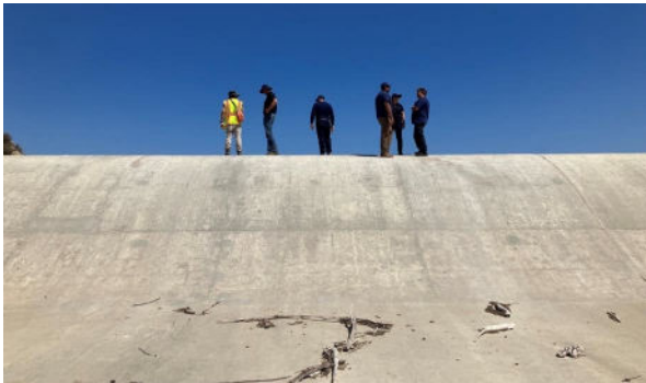
Inspection of Ogee Weir
