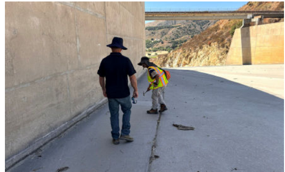
Inspection of Spillway Slab
