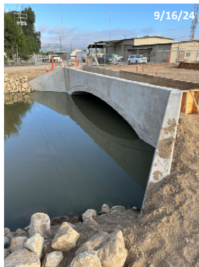
Partially Completed Bridge Replacement
