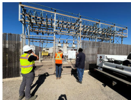
Top: DWR Site Visit, Bottom: Electrical Site Visit
