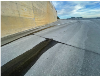
Spillway slab seepage March-April 2024.
