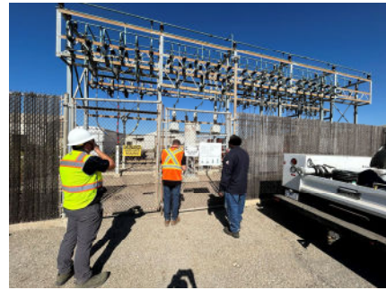
Top: DWR Site Visit, Bottom: Electrical Site Visit
