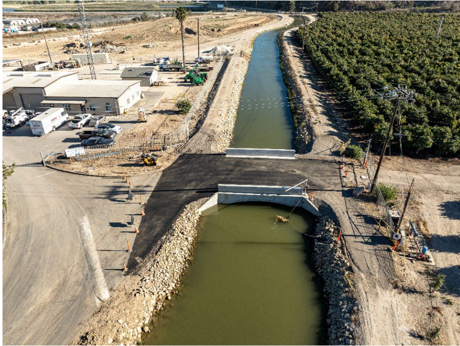
Figure 2 - Drone Image of Inverted Siphon Replacement Project (dated October 22)
