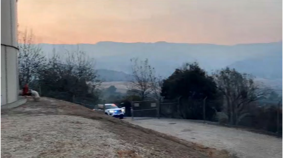
Irrigation and domestic tanks
