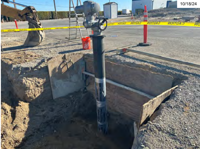
12" Valve with elevated AUMA for Pressure Relief Station
