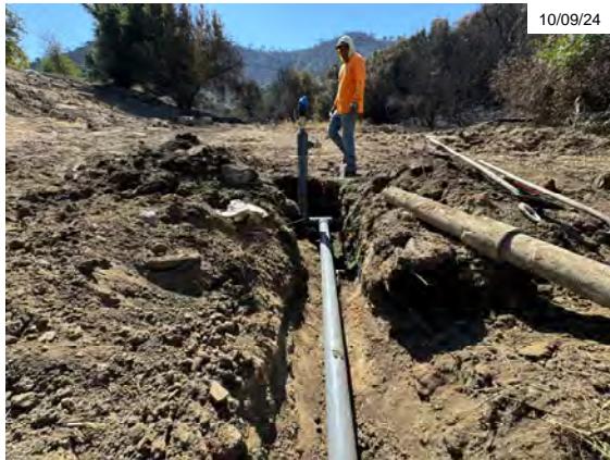
Leak Repairs caused by Felicia Fire
