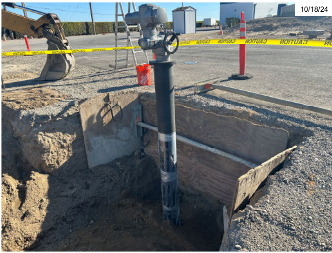
12" Valve with elevated AUMA for Pressure Relief Station
