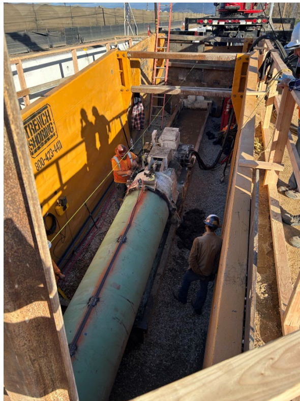
Figure 4 - Conductor Casing Pit 1 (East) Installation - Laguna Road Recycled Water Pipeline (December 13)
