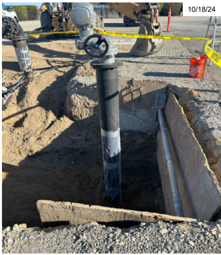
12" Valve with elevated AUMA for Pressure Relief Station
