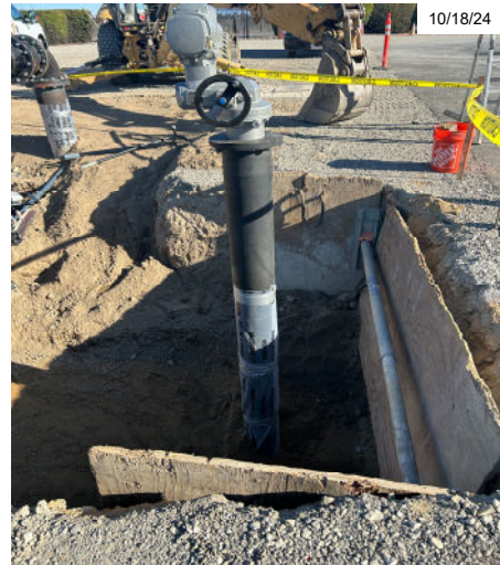
12" Valve with elevated AUMA for Pressure Relief Station
