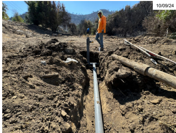
Leak Repairs caused by Felicia Fire
