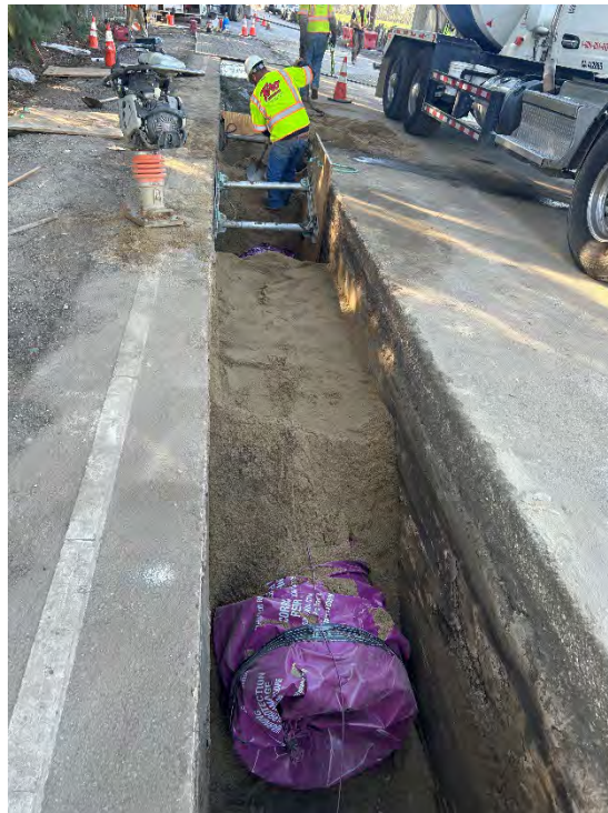
Figure 5 - 24" PVC Pipeline Installation (dated January 29, 2025)
