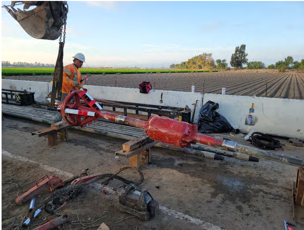
Figure 3 - 27" Reaming During the HDD Operation (dated January 3, 2025)
