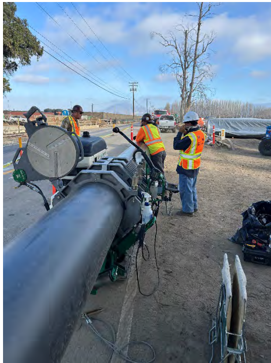
Figure 2 - HDPE Fusion Process (dated December 30, 2024)
