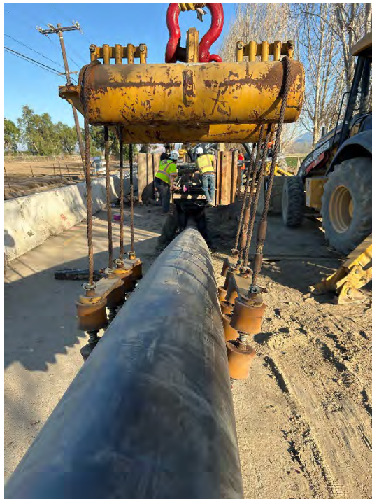
Figure 4 - 18" HDPE Pipeline Pullback During the HDD Operation (dated January 11, 2025)
