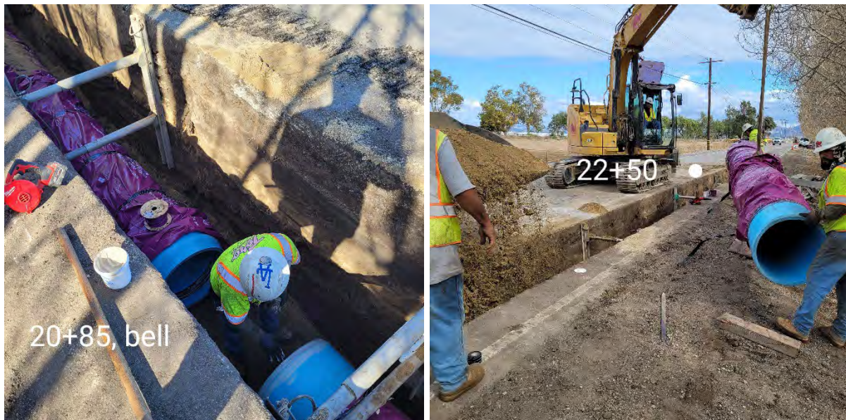
Figure 1 - Construction of 24-inch PVC Pipeline along Laguna Road (photo dated February 4).
