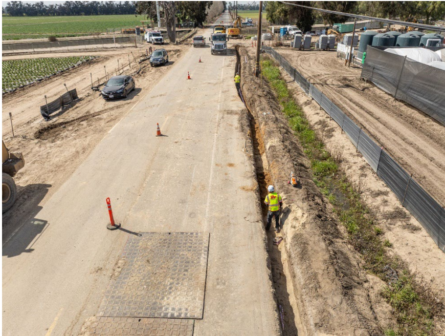
Figure 3 - 4-inch blow-off installation leading to VCWPD property on March 10, 2025
