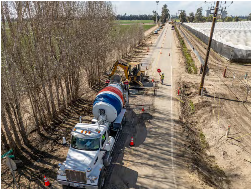
Figure 2 - Slurry backfill around meter and check valve vaults on March 10, 2025
