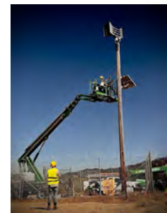
July 23, 2025 – Dam Siren Upgrade at Piru Spreading Grounds
