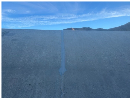
SFD Spillway Ogee Weir
