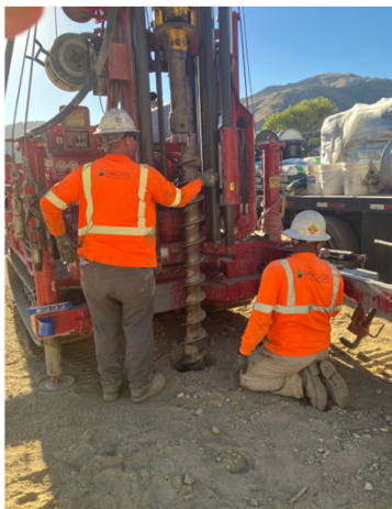
New Release Channel Drilling - November 2024
