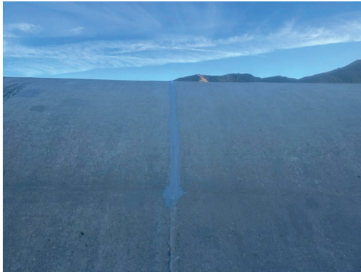
SFD Spillway Ogee Weir
