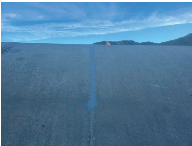
SFD Spillway Ogee Weir
