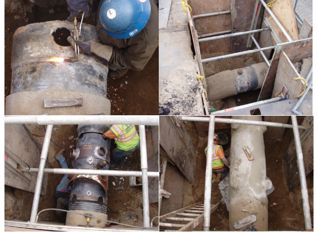
OH Repair at C Street - 2011
